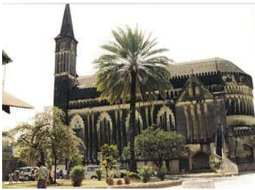
The soon to be restored Anglican Church in Zanzibar.
